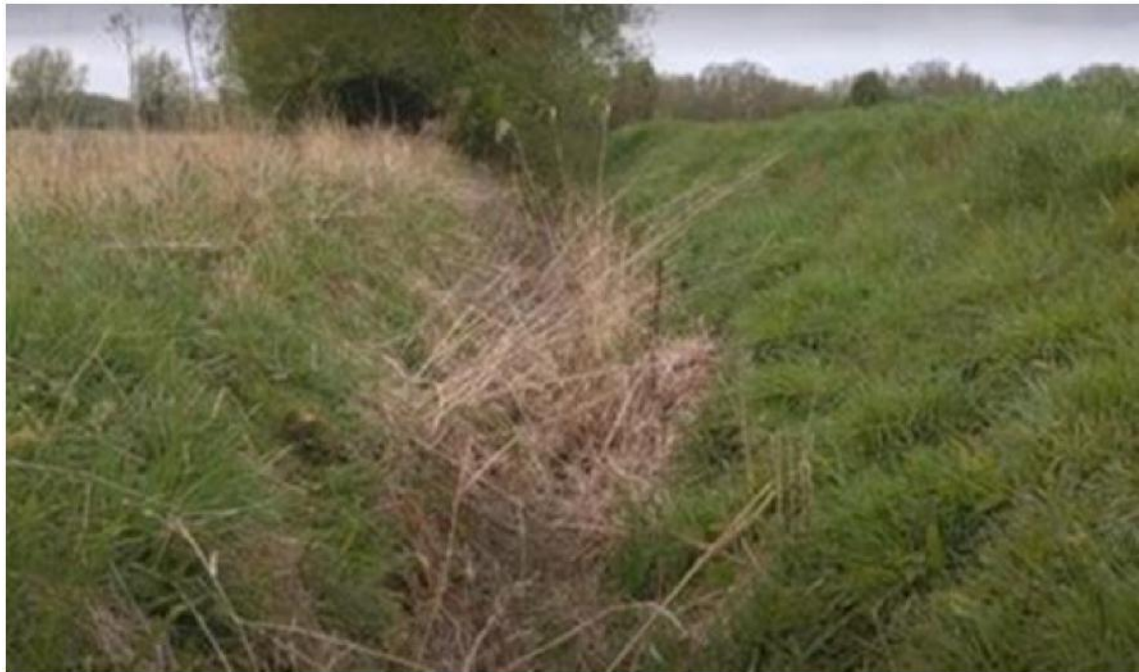
Photo 1 Existing ditch along northern boundary of Work Area 39
